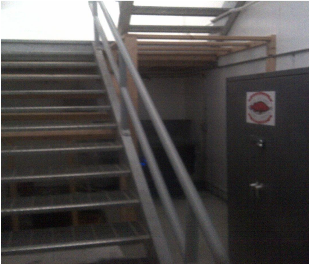
Project resource maintenance starting installation of enclosure to protect north count station PIT antenna equipment.
